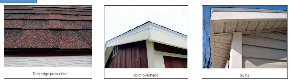
**Shingle Roof will** feature a full ½" OSB sheathing. OSB stays flat and straight and is stronger than plywood. Hclips are placed at all horizontal seams to provide extra support and ensure proper spacing between panels. All shingle roofs come with drip edge protection on the edges to prevent moisture from seeping under the shingle.
