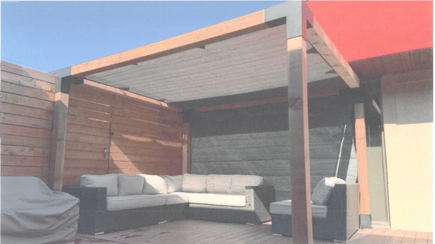
Installed Toja Grid with 6\"X6\" Western Red Cedar Beams and installed shade
